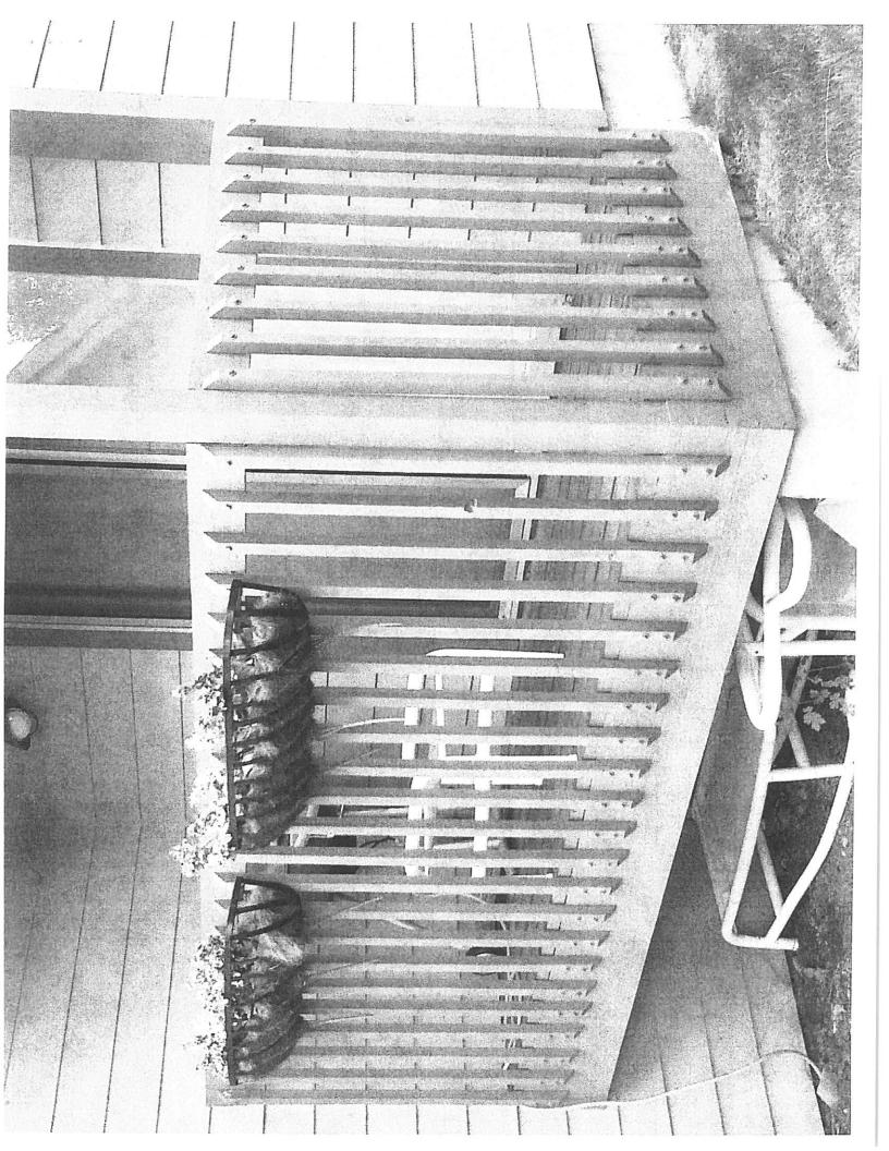
Mouse to post concreted in ground. In Makerials 2x4, siding to match Makerials-Pressure treated lumbar consisting of 4x4, 2x6 x 2x4, siding to match house and top plate lend plates painted to match house. Note top plateland plate not present. Privacy wall constructed on back patio, attached from corner of TXT
